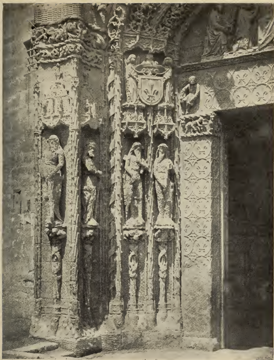
SPAIN (end of the xv Century). Detail of the façade of San Gregorio at Valladolid.
