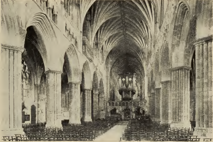
ENGLAND (XIII Century). Exeter Cathedral, the nave.
